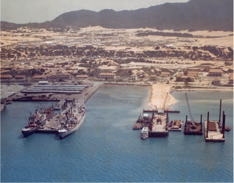
The second DeLong cargo pier was completed at Cam Ranh Bay in August 1966, and work on the third DeLong pier (to the right of the first DeLong pier) had begun.
